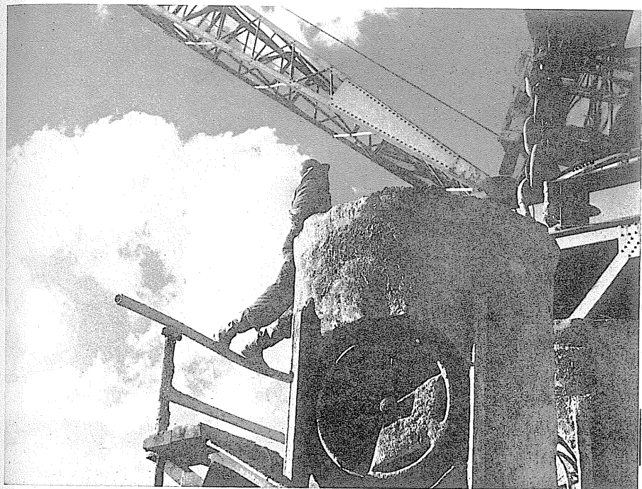
At Douglas Dam a workman hooks an 11-ton concrete bucket to the handling crane.
